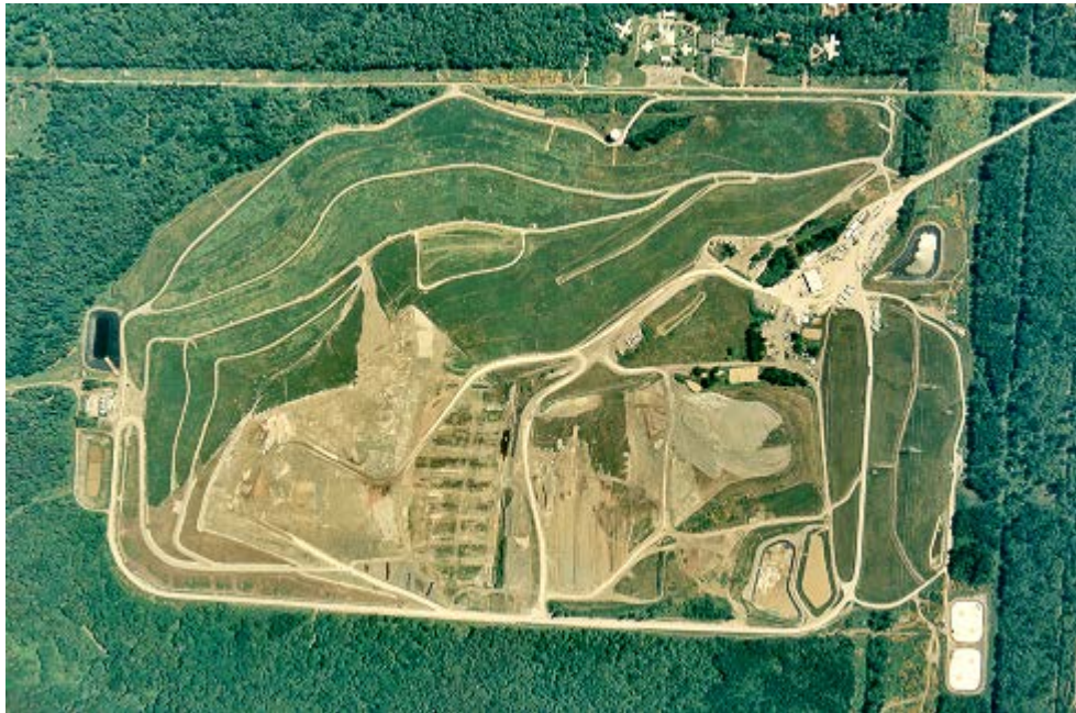
Aerial View of Cedar Hills Landfill – May 1998
